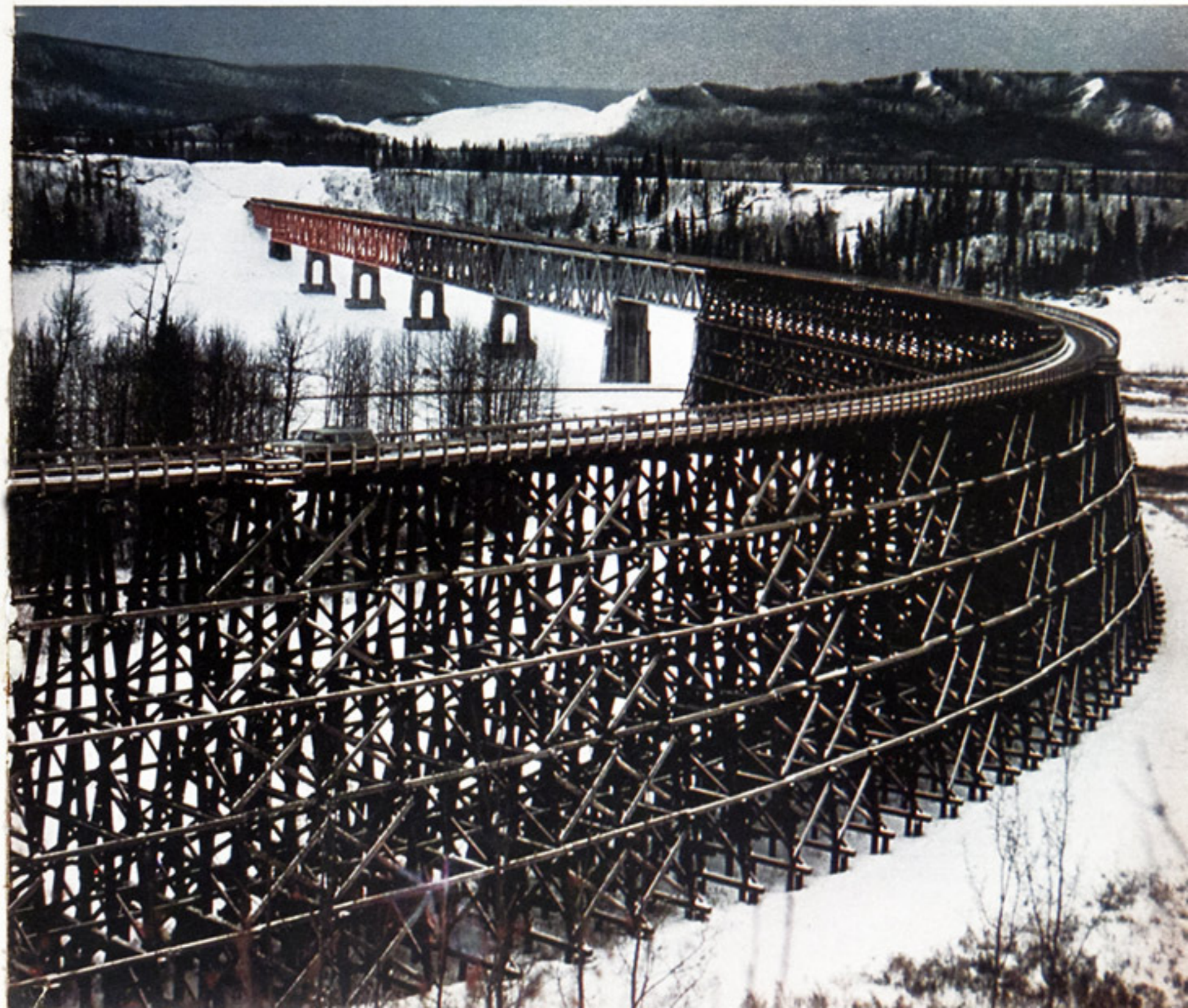
This converted railroad trestle over the Peace River stands in for a highway bridge that collapsed in 1957.
