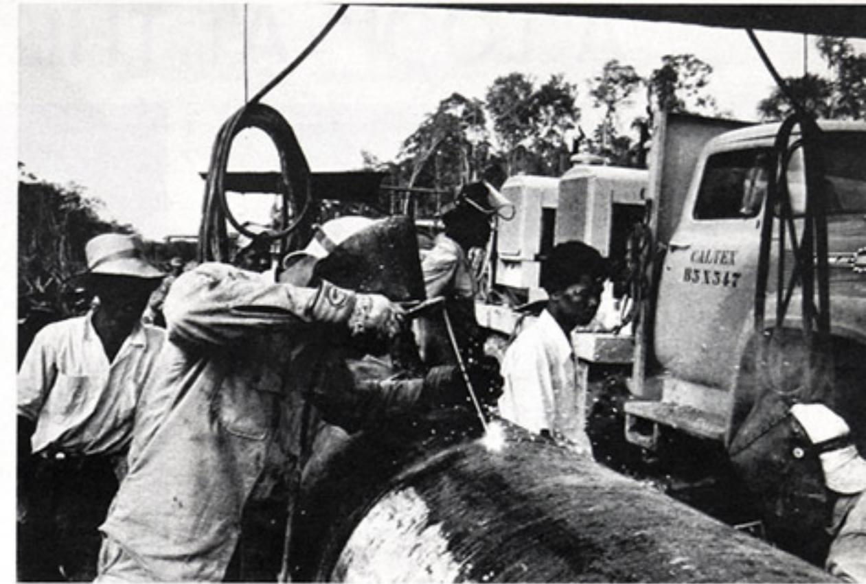
**LAYING PIPELINE**, two Texas welders seal joint in a section of the new 30-inch line that will carry the oil from the rich Duri fields to new deepwater
